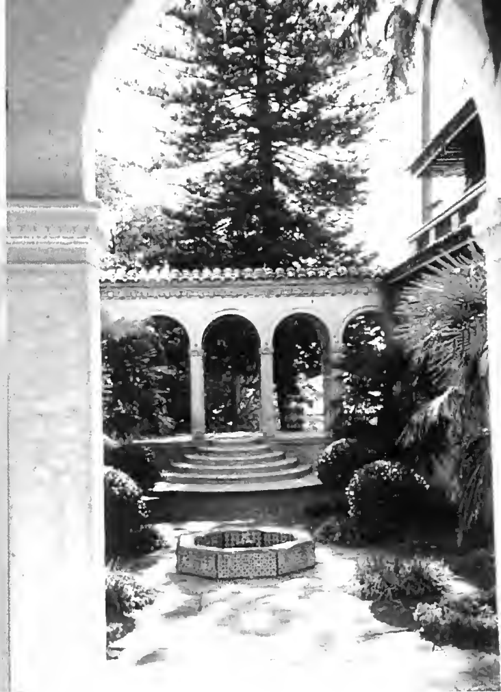
The Cloister at Boomerang, Billyard Avenue, Elizabeth Bay, 2001. Photo: Stuart Read.
